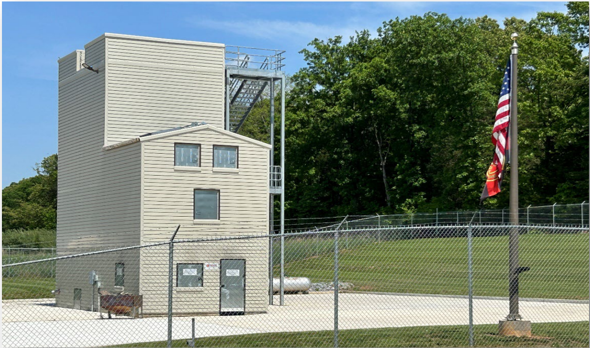
New Fire Tower Training Facility
